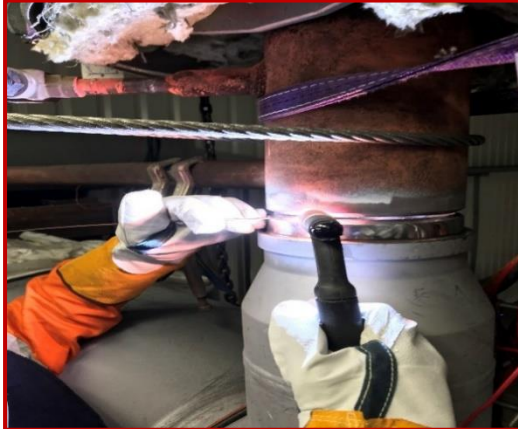
Inspection of 24" Root Run & Cap
